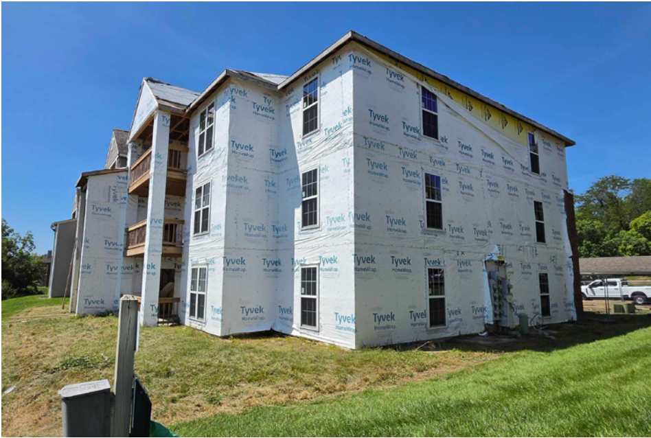
Image: Multi-family building currently under construction in Cincinnati, OH
